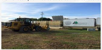
Thermal desorption involves the excavation and on-site treatment of impacted soil using a closed-loop steam desorption unit. Impacted soil is mixed and blended with lime in-situ before being loaded into the treatment system in lifts of approximately 15 cubic yards. Superheated steam is forced through the impacted soil to volatilize adsorbed VOC constituents. Both the steam and VOC vapors are then recovered from the treatment
